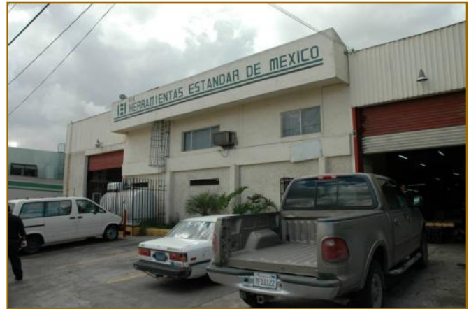
Production Facility, Tijuana MX
